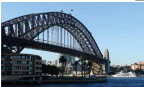
Sydney Harbour Bridge
