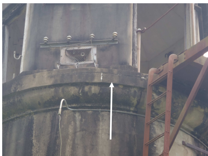
Figure 15 View of cracking (shown arrowed) to string course of pumping station
