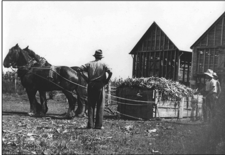
Figure 13: Horses pulling a loaded sled in front of timber-framed sheds on River Farm c1920s. The sheds are characterised by an internally fixed, timber slat lining. A shed of the same design is extant (P320 UWS Archives)
