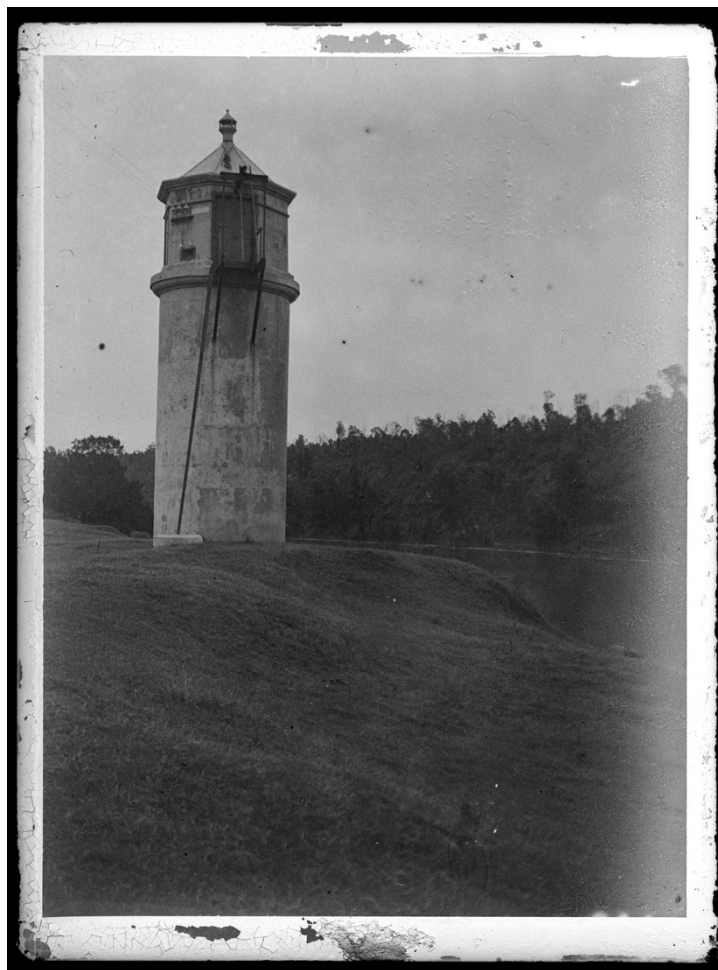
Figure 19: The reinforced concrete tower of the 'pump well' or pumping station at River Farm in 1914 (Perrett, ON 216, ML SLNSW)
