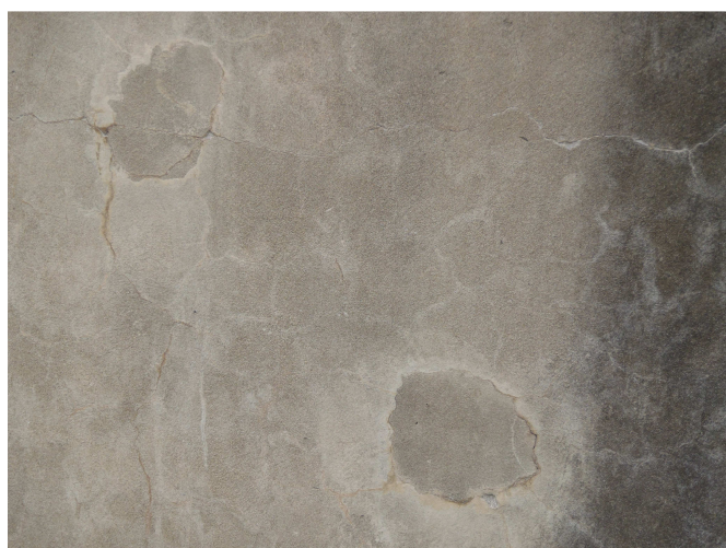
Figure 16 View of previous patch repairs to pumping station
